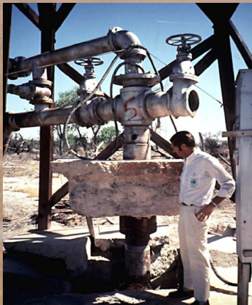
Left: Effects of subsidence at water well head.
