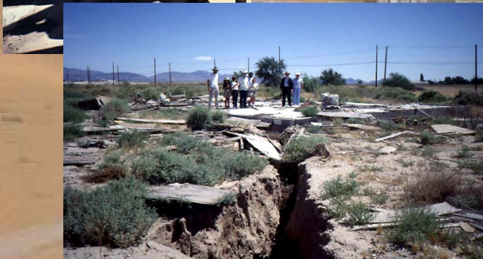
Below: Fissuring due to subsidence caused by oil exploitation.
